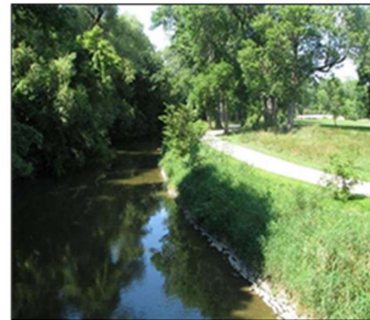
View looking north from footbridge at east bank. Conditions = high grass and little sign of erosion.
