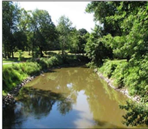
View south, downstream, from the footbridge. Both banks are in good condition.
